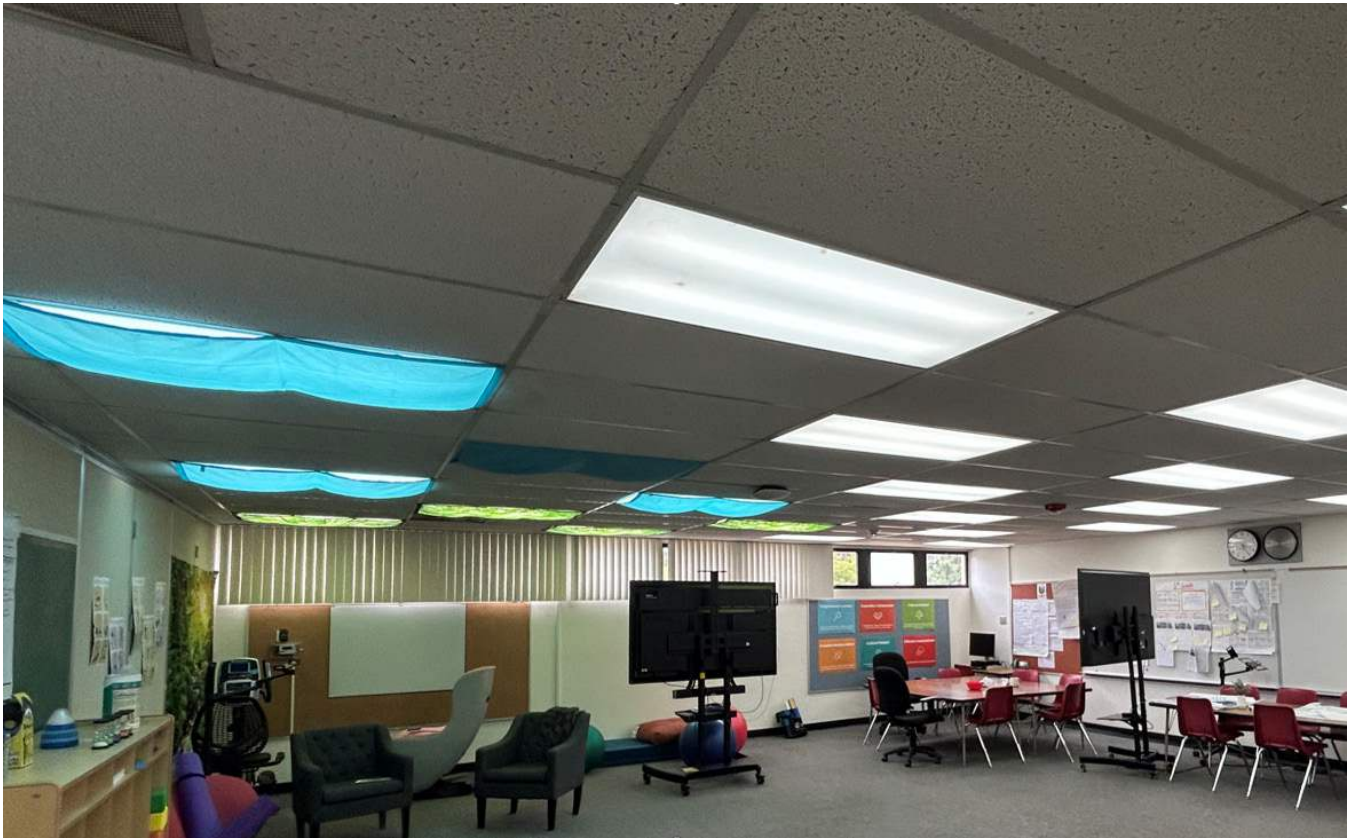
Figure 7. K-5 classroom with modified lighting to support diverse learning activities. Desk plane illumination is 735 lx, while vertical plane melanopic EDI is 176 (70% of blue sky criterion).
